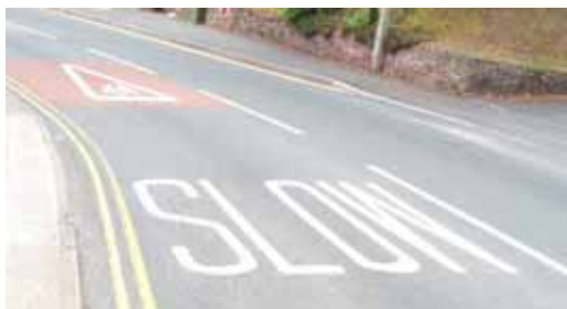
DfT Approved Road Marking on Coloured Surfacing Oldway Primary School
